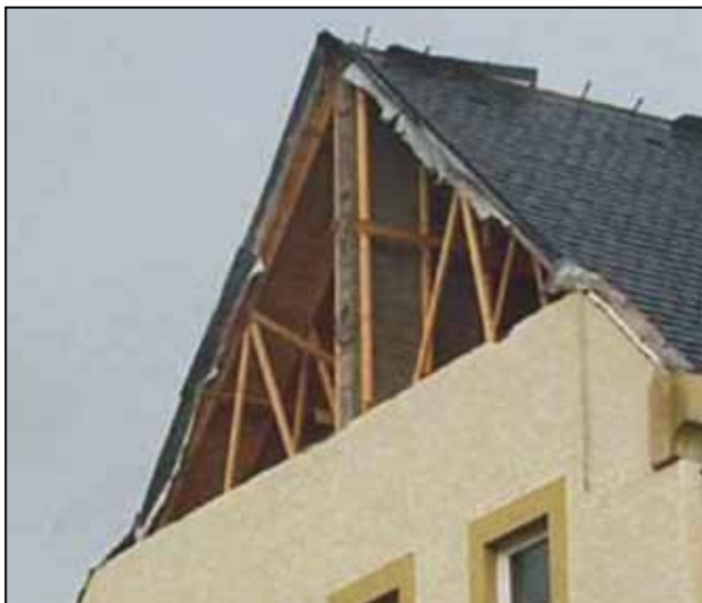
Fig 3.9: Gable wall failure
