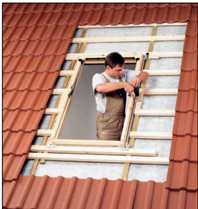
Fig 5.10: Securing the frame
