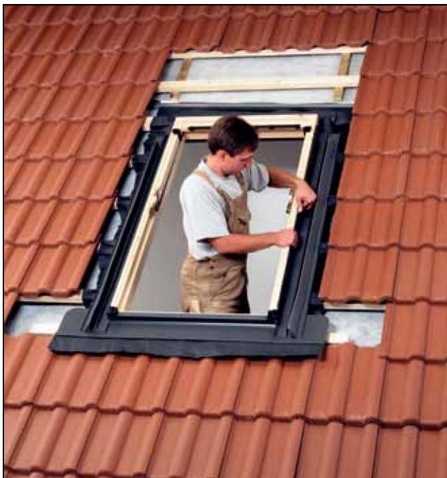
Fig 5.11: Installation of weatherproofing arrangement
