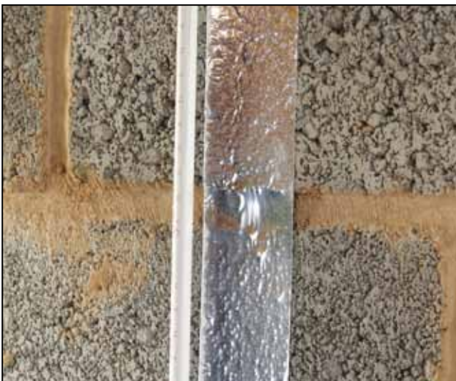
Fig 11.2: Positions for metallic tape by plastic pipes
