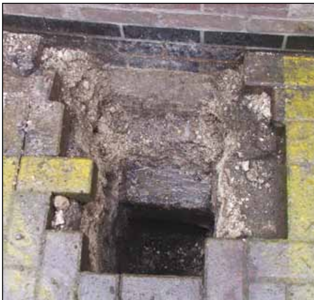
Fig I 3.5: Trial hole for foundation inspection
