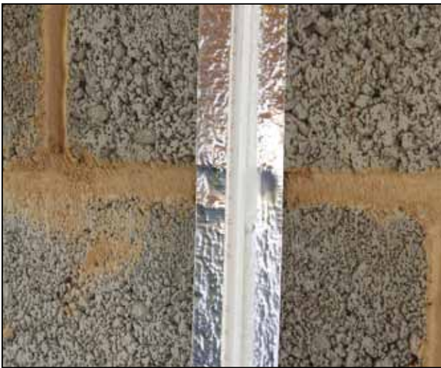
Fig 11.1: Positions for metallic tape by plastic pipes
