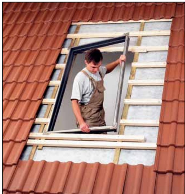
Fig 5.9: Inserting the support frame
